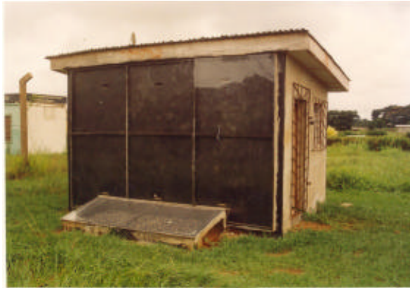
Fig. 1: Trombe wall poultry chick brooding house
